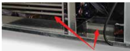
Drain pan heating element for condensation evaporation
