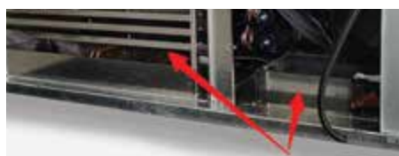
Drain pan heating element for condensation evaporation
